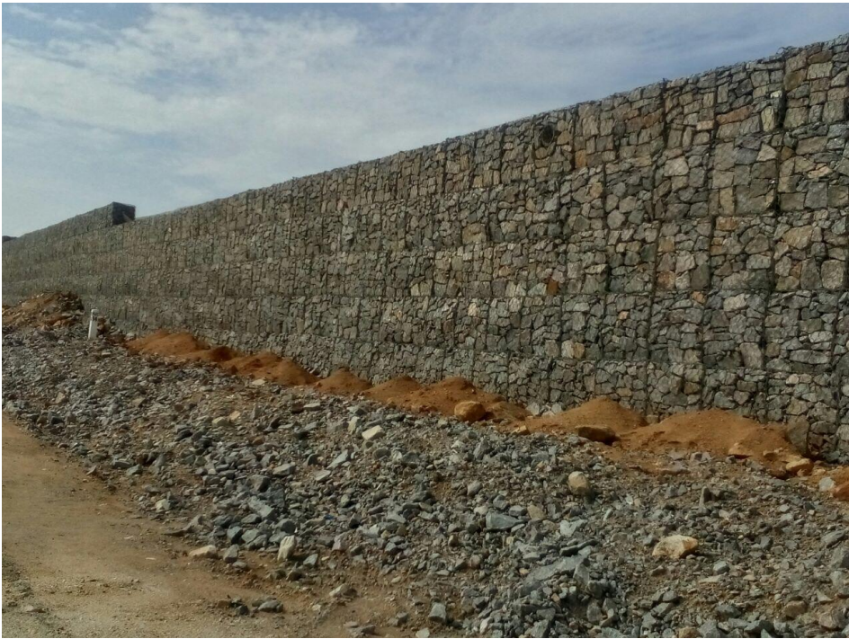
6 meter height wall constructed for retention for road structure
