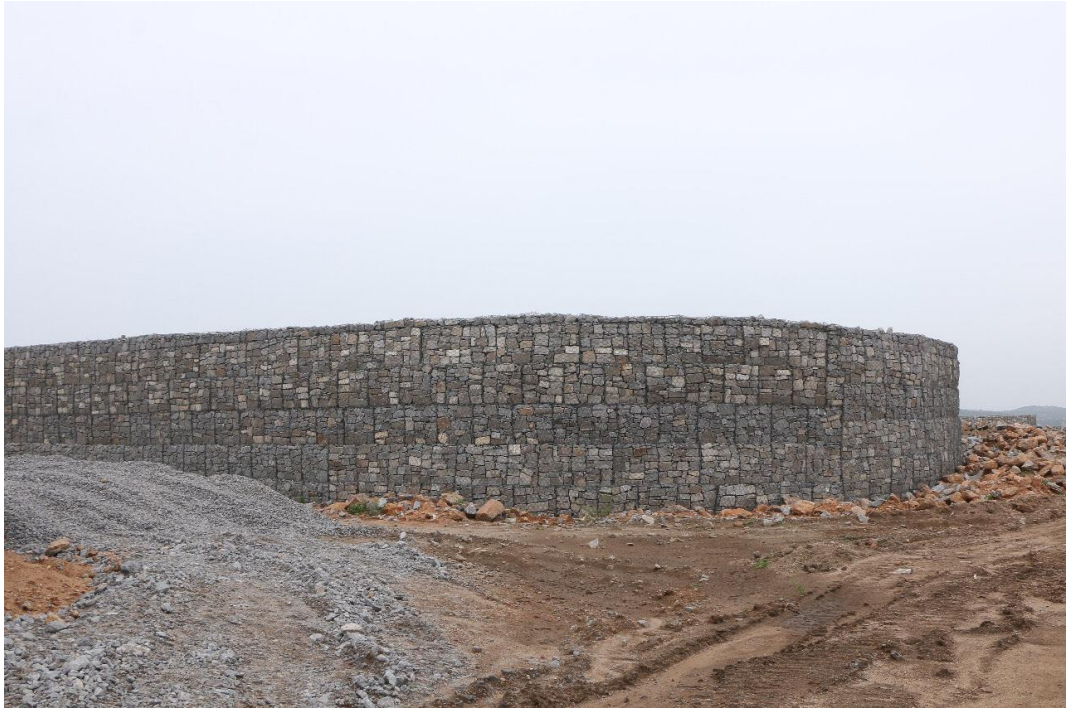
Gabion wall during construction
