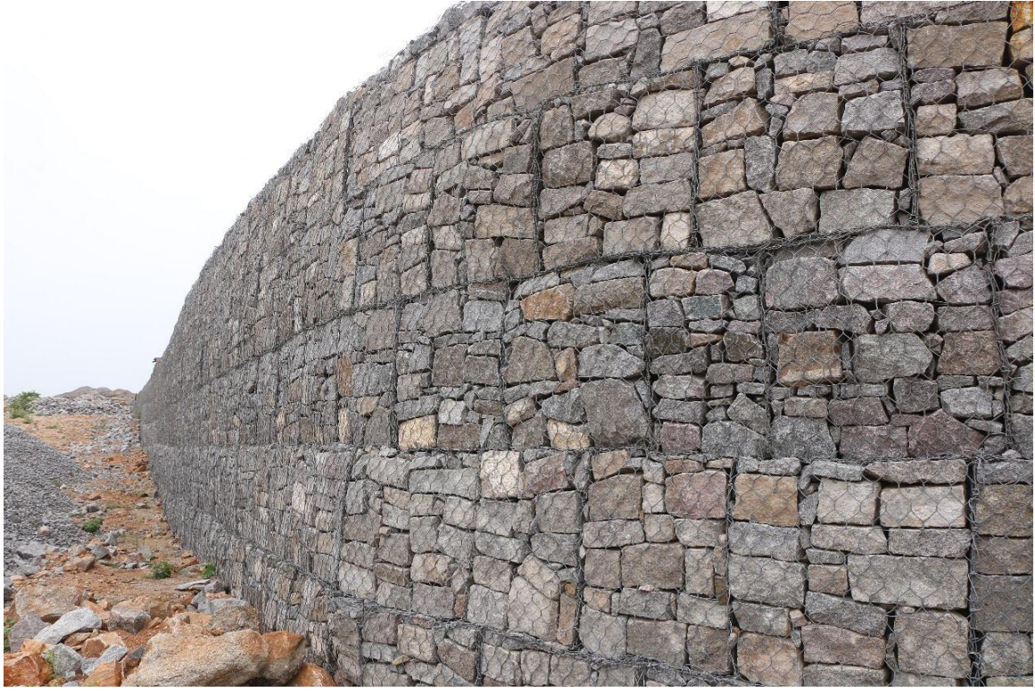
Gabion wall close up at curved surface
