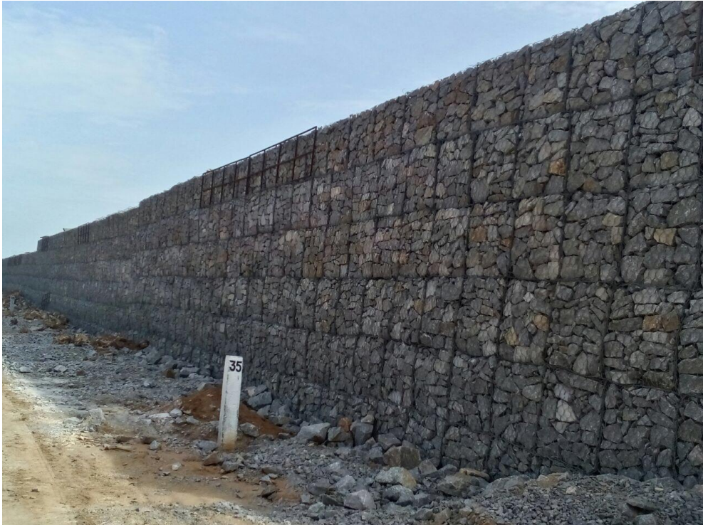
6 meter height wall constructed for retention for road structure
