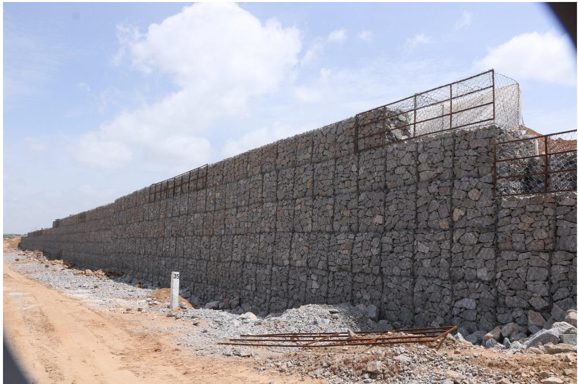
Gabion wall during construction
